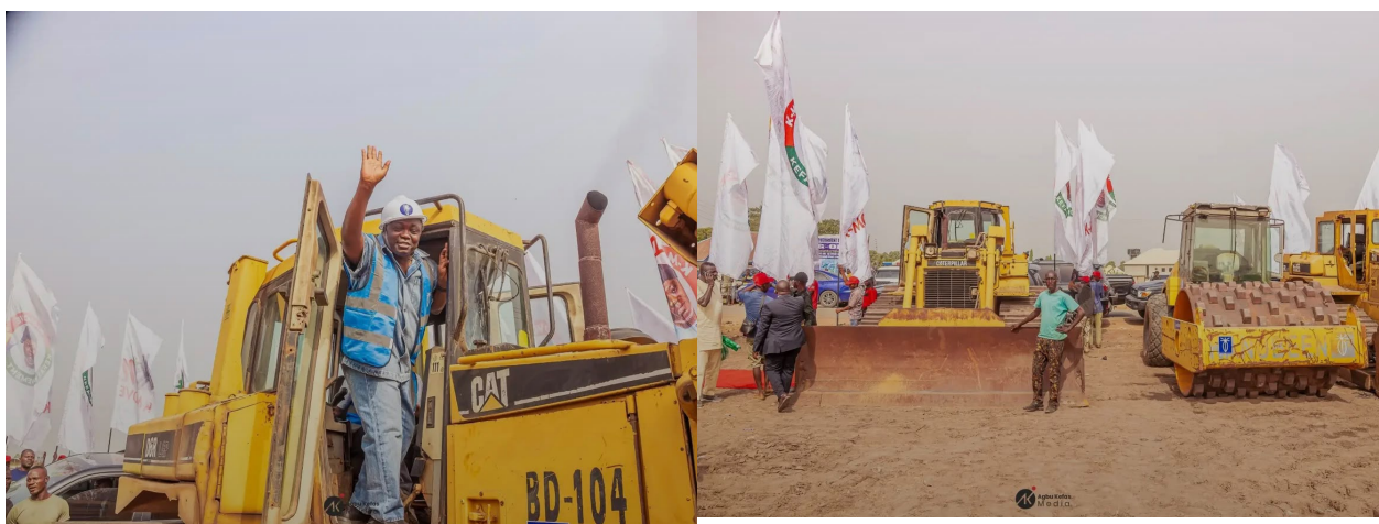
Governor Kefas waves from atop a CAT bulldozer during the flag-off of a major road construction project in Taraba State.
